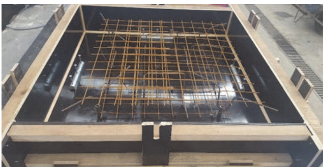
Figure 3. Reinforcement in concrete slabs
