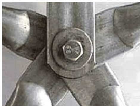
Figure 3. Several solutions of steel geodesic dome nodes [5]
