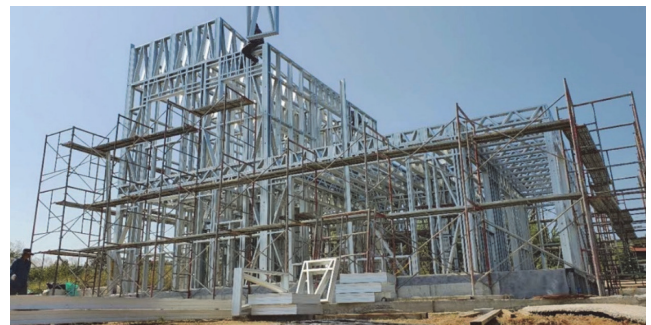
Figure 9. Construction of an urban villa with a lightweight panel construction system [19]
