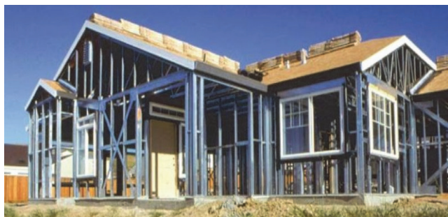
Figure 1. House with a steel structure [2]
