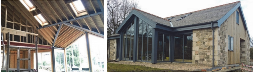
Figure 7. Family house built in a combination of steel and wood [16]
