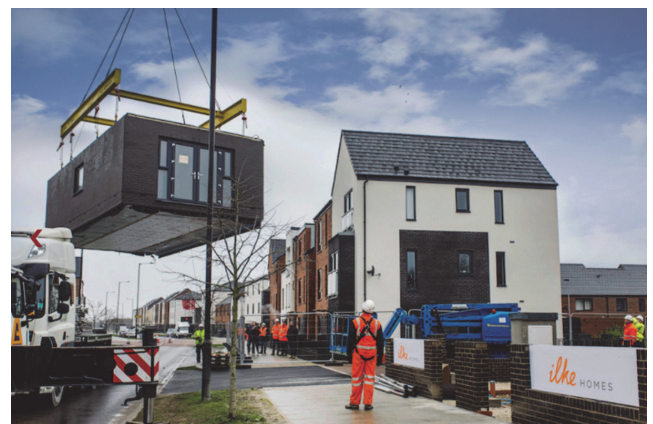
Figure 13. Positioning the steel module of the house [24]
