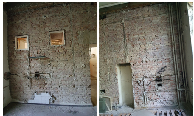
Figure 25. Typical masonry walls with openings and installations
