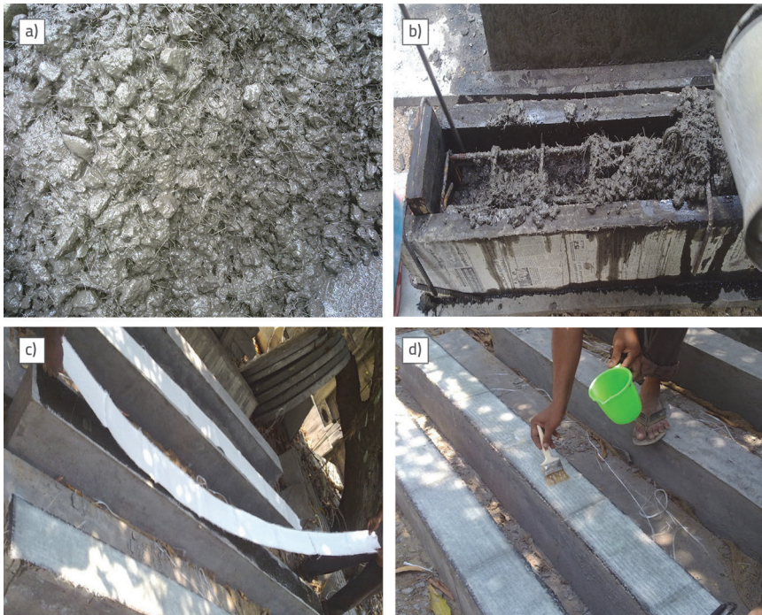
Figure 2. Beam casting and strengthening in progress
