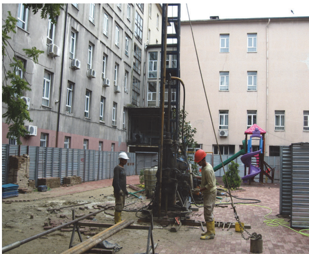
Figure 11. Cement grouting for ground strengthening
