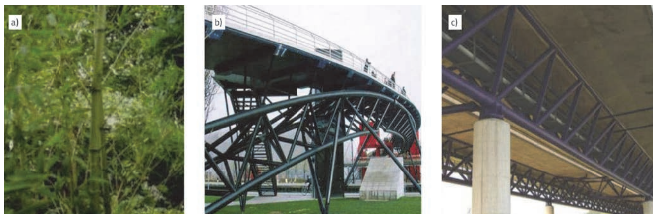
Figure 1. Application of circular hollow section (CHS) member [1]: a) Bamboo; b) Aesthetically appealing; c) Bridge with circular girder
